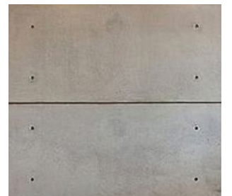
6. PANEL FORMED CONCRETE
