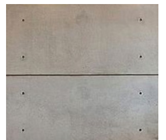
6. PANEL FORMED CONCRETE
