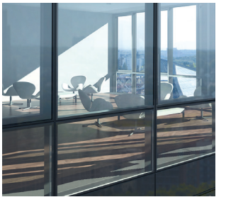
2. CURTAIN WALL - HIGH PERFORMANCE GLAZING
