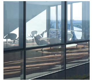
2. CURTAIN WALL - HIGH PERFORMANCE GLAZING
