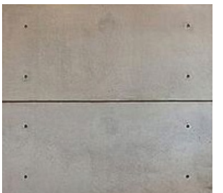
6. PANEL FORMED CONCRETE
